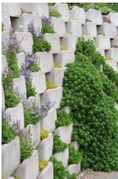
Vegetated retaining wall systems are an aesthetically pleasing choice for typical site retaining wall installations. Vegetated retaining walls transform hardscape into landscape while providing for storm water retention, heat island mitigation and erosion control. Vegetated retaining wall systems require less concrete and labor, and can offer greater cost savings depending upon project conditions.
